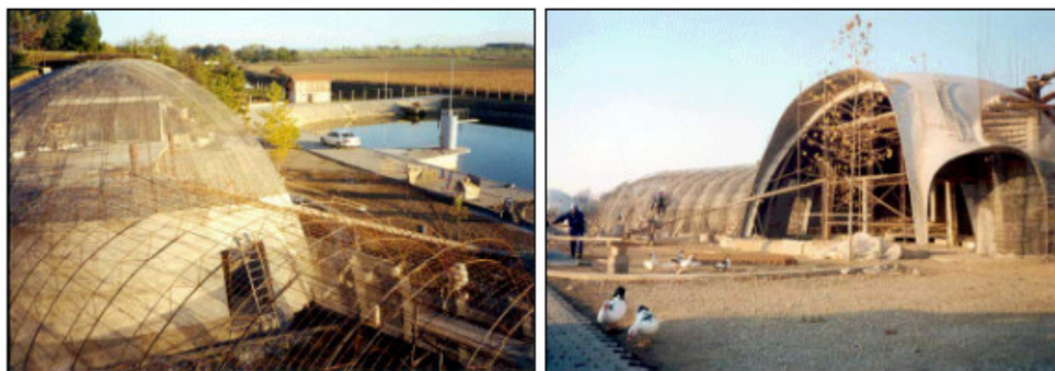
Figure 1. Sample ferrocement structure - solar home. (Courtesy: www.ferrocement.com )
