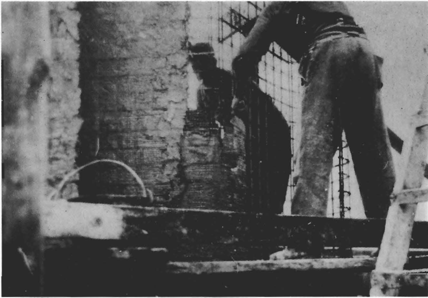
Fig. 6 Picture of construction site during mortar laying (Archivio Antonio Nervi)
