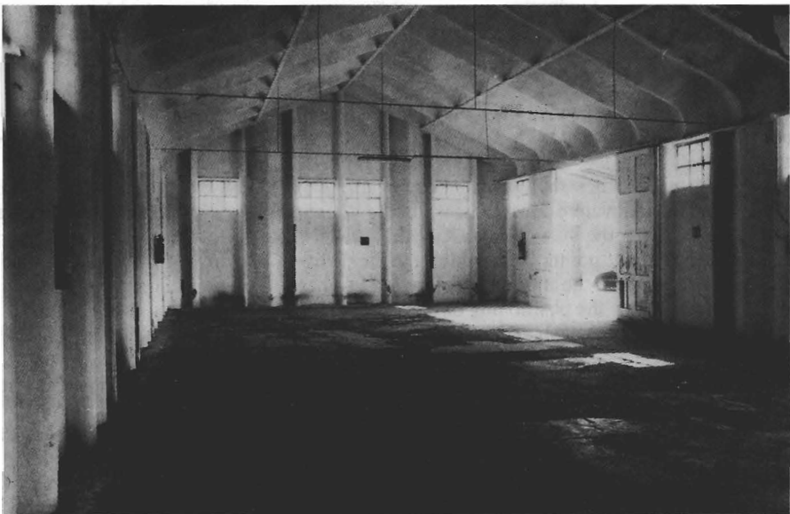
Fig.7 View of the interior of the storehouse today
