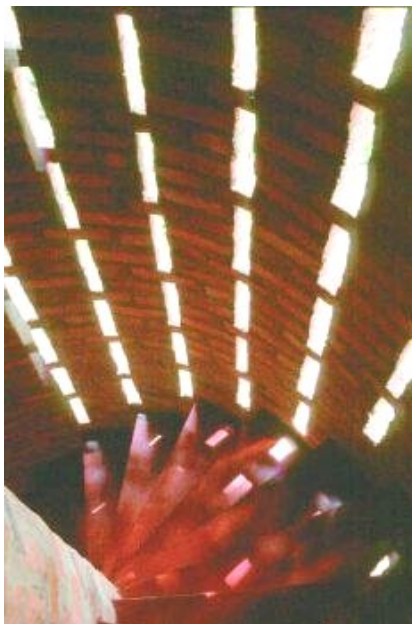
A stairwell in a residence in trivandrum has a perforated brick wall creating
